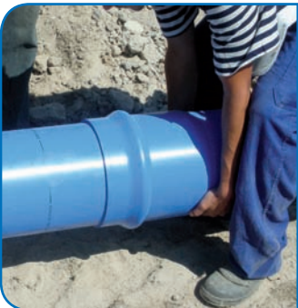
Align the pipe and place the spigot end inside the socket or bell.
