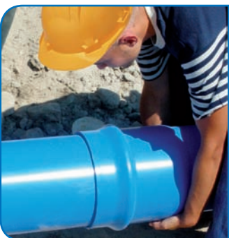
Firmly push the free end into the other pipe. Introduce until the end marked is no longer seen.
