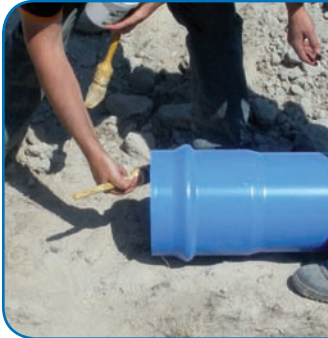
Apply lubricant on the chamfer of the spigot end and in the rubber ring joint.
